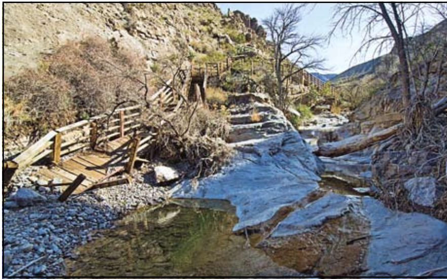
A 500-year flash flood sent a 20-foot wall of water down Dog Canyon in 2008, destroying the boardwalk at Oliver Lee Memorial State Park.
