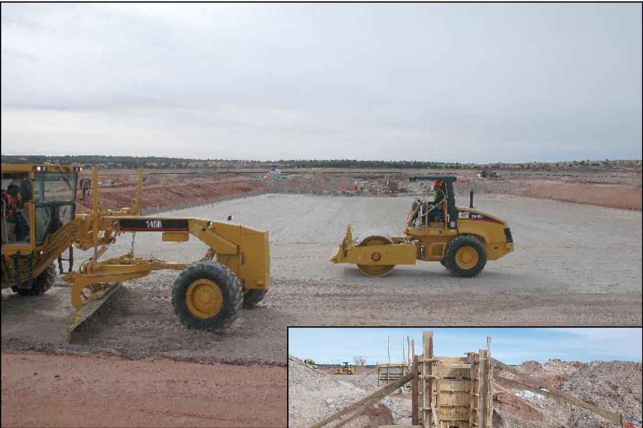
Mike Sloane, Chief of Fisheries for the Department of Game and Fish, and Rock Lake Hatchery Manager Roddy Gallegos inspect forms for concrete water gates (right) that will allow hatchery crews to capture warmwater fish raised in one-acre ponds (above). Construction of the first phase of the $8 million hatchery was expected to be completed this spring.
