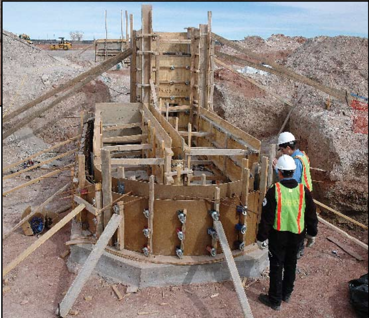
Mike Sloane, Chief of Fisheries for the Department of Game and Fish, and Rock Lake Hatchery Manager Roddy Gallegos inspect forms for concrete water gates (right) that will allow hatchery crews to capture warmwater fish raised in one-acre ponds (above). Construction of the first phase of the $8 million hatchery was expected to be completed this spring.
