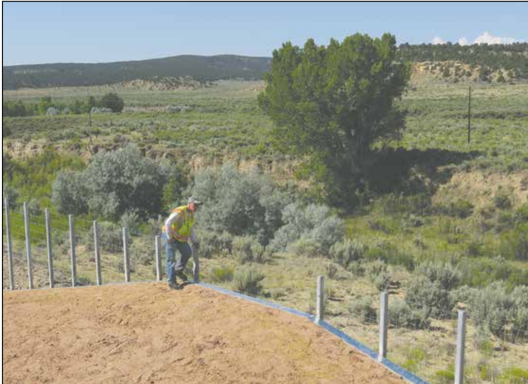
Above: Jim Hirsch of NMDOT Environmental Bureau inspects a newly constructed wildlife escape ramp on U.S. Highway 550 south of Cuba. Department photo by Mark Watson.
